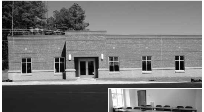
Exterior and classroom in Oconee QuickJobs Center
